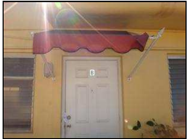
2.4 Picture 6 12207 - B - Not secure to building.
