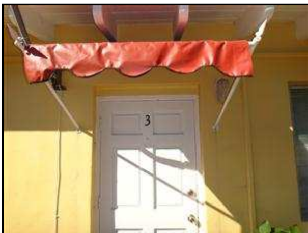
2.4 Picture 3 12209 - 3 - Not secure to building.
