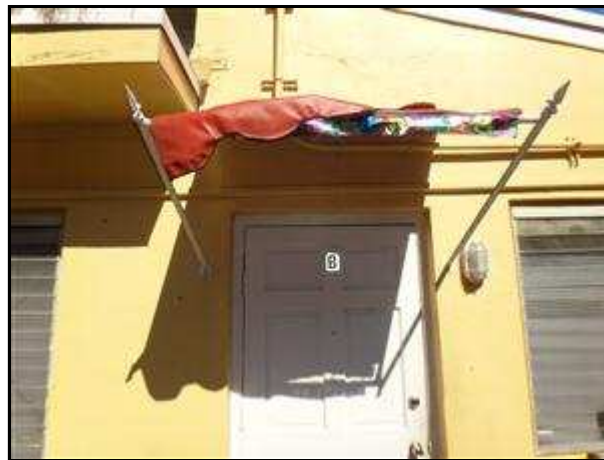
2.4 Picture 7 12205 - B - Not secure to building.
