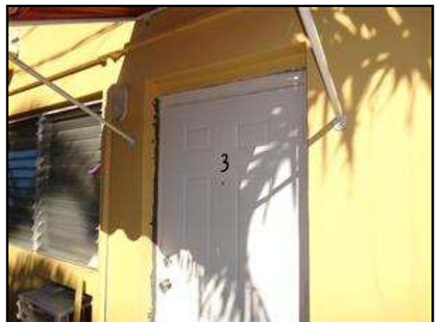
2.4 Picture 4 12211 - 3 - Not secure to building.
