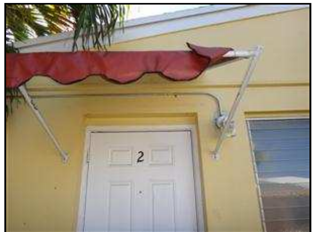
2.4 Picture 2 12211 - 2 - Not secure to building.
