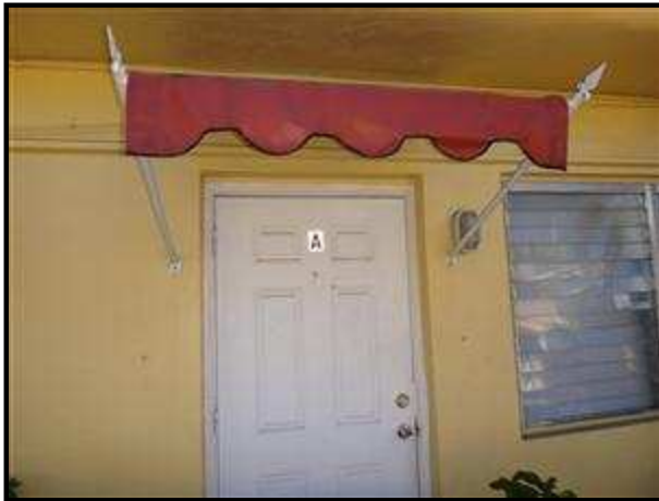
2.4 Picture 5 12207 - A - Not secure to building.
